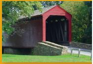
utilizes multiple king post trusses covered with clapboard. It was rebuilt after an arsonist's fire nearly destroyed it in 1991. The bridge is 90 feet in length and 12.2 feet high.
